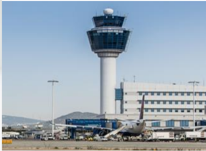
ATHENS INTERNATIONAL AIRPORT
